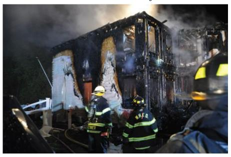
(2) This modern house had extensive and rapid fire envelopment outside because of the combustible siding, insulation, and sheathing. Note the collapse of the truss roof, which occurred early in the fire.
